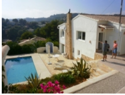
East side of house + pool
