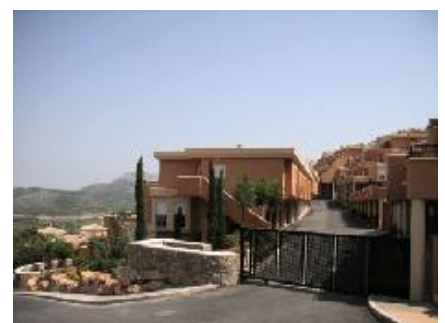
Electric entrance gate
