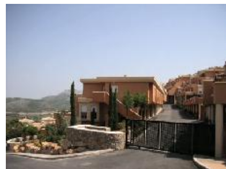
Electric entrance gate
